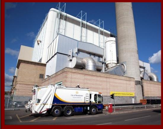
Residual waste (the waste that can't or shouldn't be recycled) is delivered under a long term contract to South East London Combined Heat and Power, a waste fired power station in Deptford. Here waste is burned to generate green electricity for around 50,000 London
